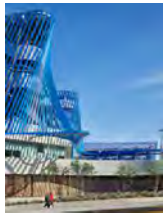
ABOVE LEED and envision certified Angle Lake Transit station
