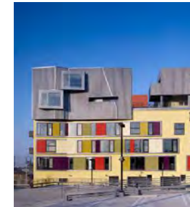
ABOVE A new two story addition of market rate housing on top of the existing 1920s historic warehouse structure.
